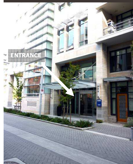
Figure 13: Principal entrances are clearly identifiable and articulated at the street frontage.
