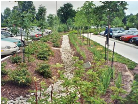
Boulevards in parking areas should incorporate soft landscape materials and shade trees with design elements and systems that mitigate storm water run-off.
