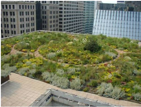
Green Roofs ameliorate the urban heat island effect and support natural habitat.
