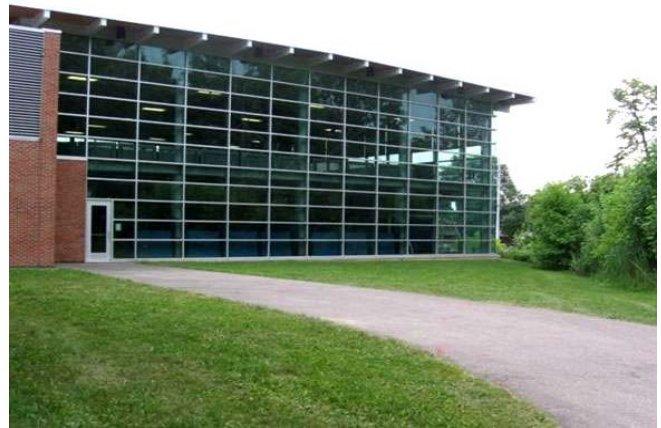
Figure 3.0.3 Natural surveillance from the community centre gymnasium to an adjacent woodlot
