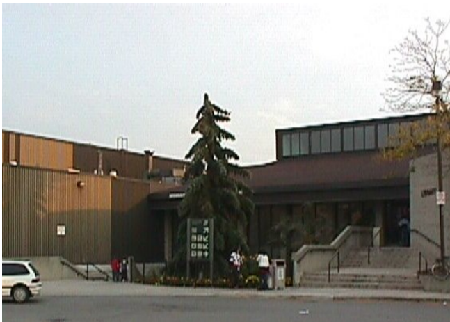
Figure 4.0.3 Before —Hidden entranceways due to the location of signage, landscaping & walls with obstructed views
