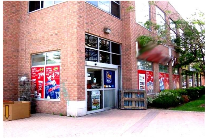
Figure 3.1.2 Not Preferred —Excessive signage in the windows limits natural surveillance opportunities to both the exterior and interior spaces
