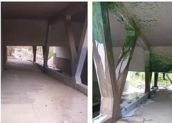
Figure 4.3.3 Before—The area under the bridge is vulnerable to graffiti; After—Murals create a sense of ownership to the space
