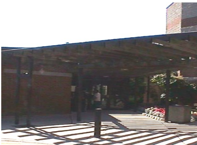
Figure 4.3.1 Before — A pergola & recessed entrance at the Malton Community Centre limits natural surveillance opportunities
