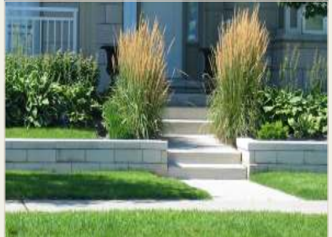
Fig. 1.2.1-7: Terraced retaining walls and landscaping.
