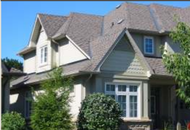
Fig. 3.3.1-2: Excellent Roof Design—a complex, varied and well composed roof form adds interest.
