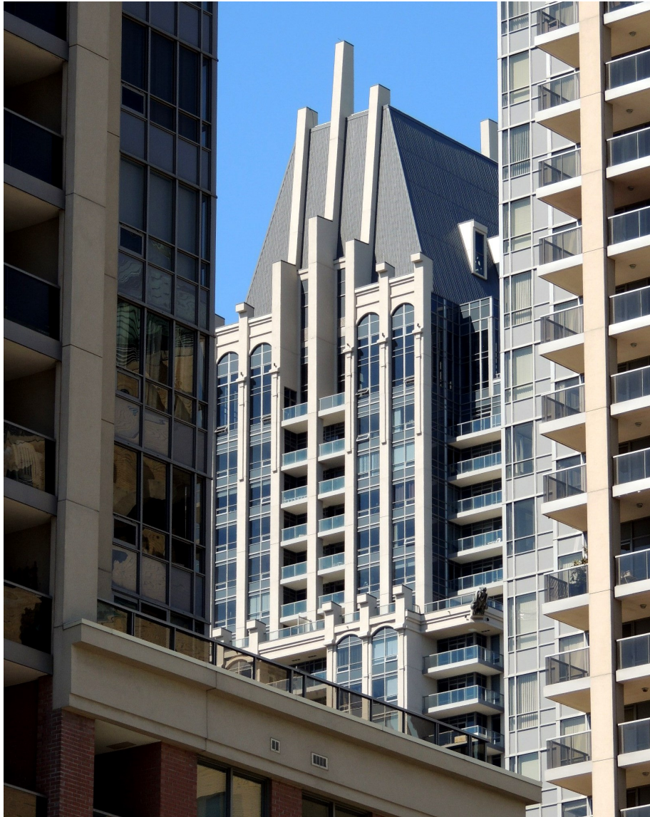
Roof Top Equipment as an integral part of the building design
