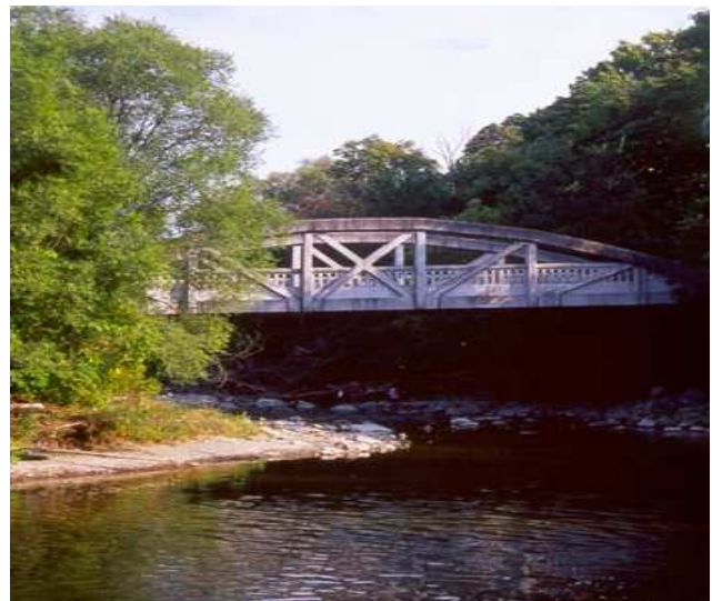
Figure 9-14: The Middle Road Bridge, located at the eastern end of Sherway Drive at the Etobicoke Creek, was built in 1909 and was the first concrete bow bridge of its kind in Canada.
