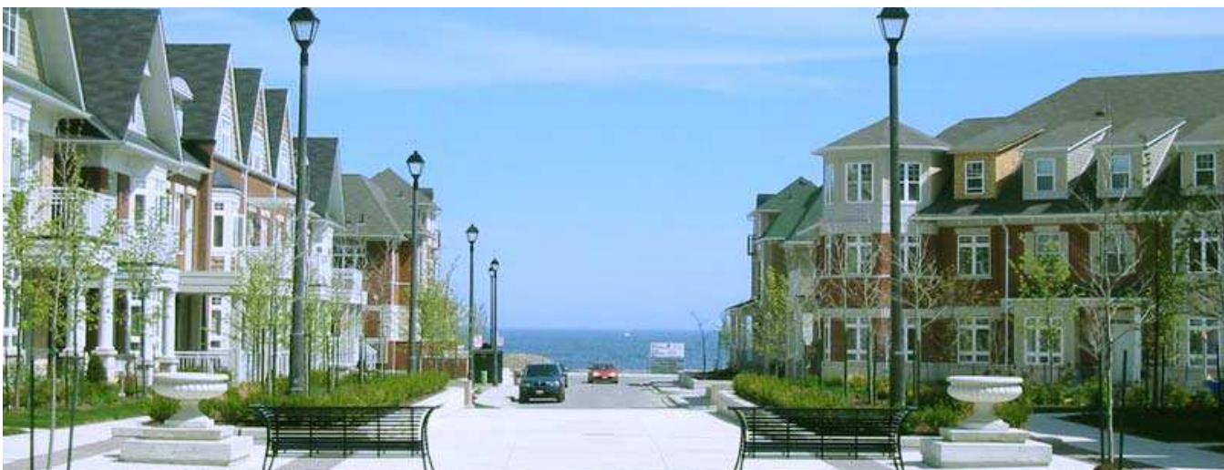
Figure 9-20: Views to Lake Ontario add value, provide a sense of orientation and preserve Port Credit's identity as a waterfront community.
