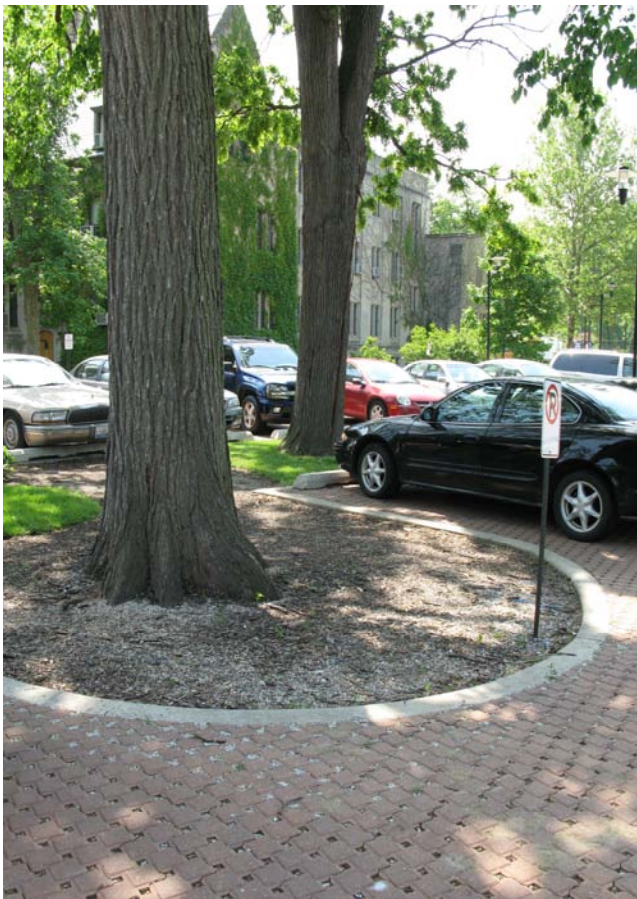
Figure 9-33: Permeable paving is used to enhance tree preservation efforts and to promote stormwater infiltration at Dominican University, in River Forest, Illinois.
