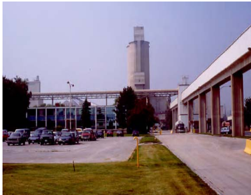
A defining aspect of Southdown's character is its industrial heritage (shown above: the St. Lawrence Cement Company).
