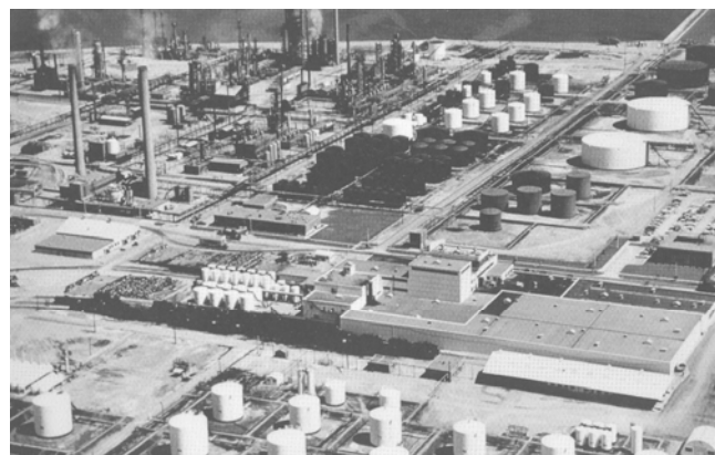
The British American Oil Company commenced building its facilities in 1944 at the edge of Lake Ontario.
