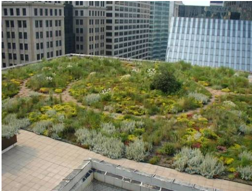
Green Roofs ameliorate the urban heat island effect and support natural habitat.
