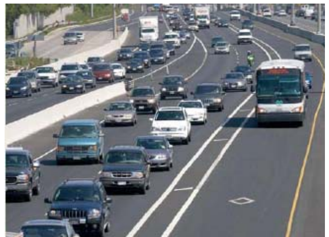
Figure 8-8: High Occupancy Vehicle (HOV) lanes such as those on Highway 403, encourage people to carpool or take transit.
