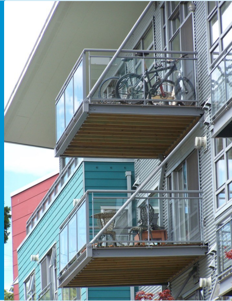
Figure 101 — Balconies should be designed so that they are part of the building rather than added onto the building as an afterthought.
