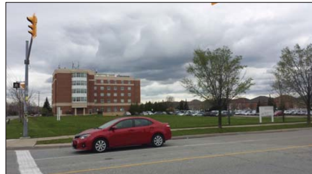
Image of existing conditions facing south from Father D'Souza Drive
