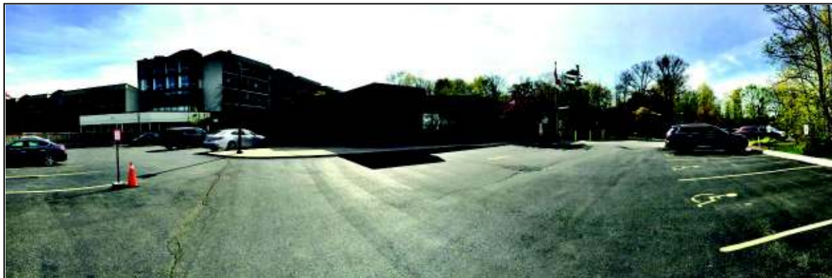
Image of existing conditions
