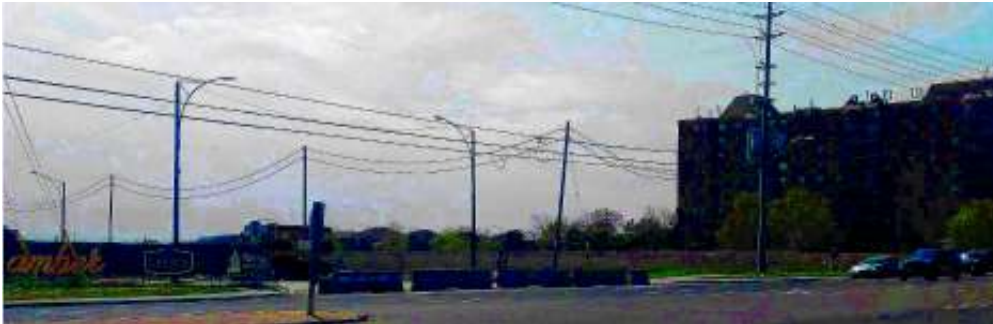
Above: Image of existing condition on the subject property, looking northwest (across Hurontario Street)
