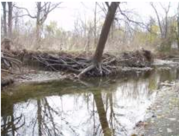
Figure 6-13: Erosion can result in serious danger to property, people, water resources, vegetation and infrastructure. Adherence to development standards and policies reduces these dangers and protects life and property.
