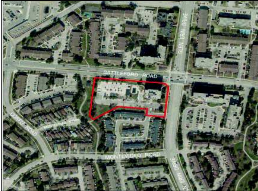
Aerial photo of subject lands
