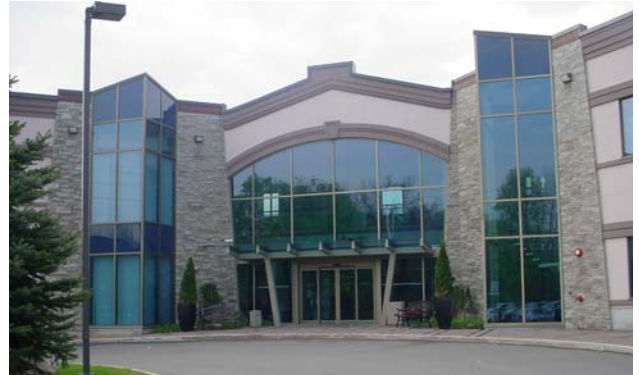
Figure 8: Existing low-rise office building.
