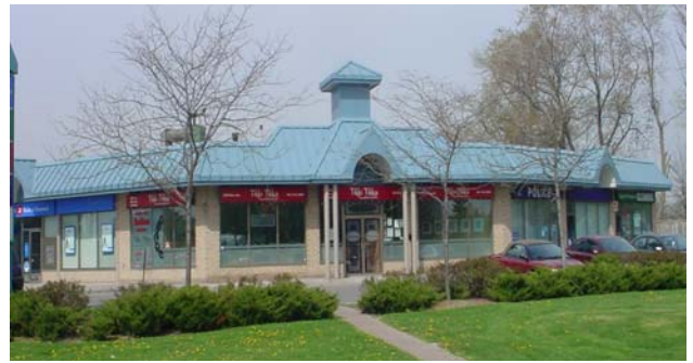
Figure 7: Northwest corner of Royal Windsor Drive and Southdown Road.
