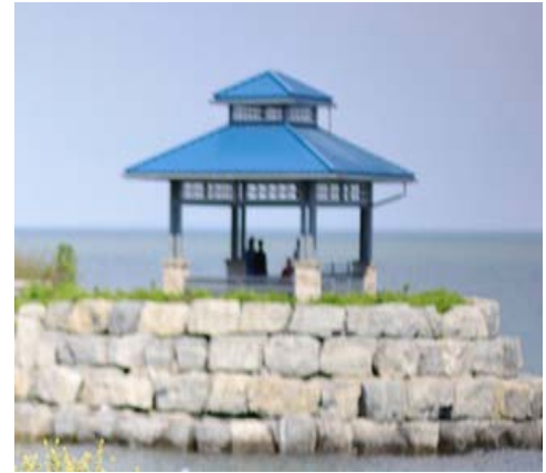
Figure 18: Provision of public access to the waterfront and protection of views to Lake Ontario are important components of Port Credit.
