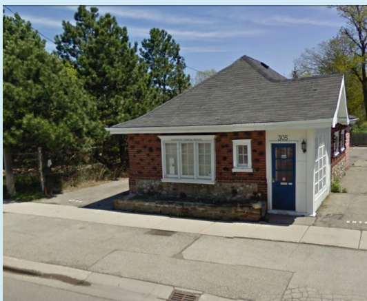
Figure C48 — 305 Lakeshore Road West Designated
