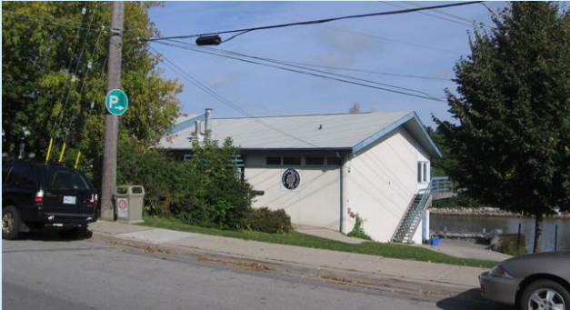
Figure B23 — Image of the Riverside Precinct
