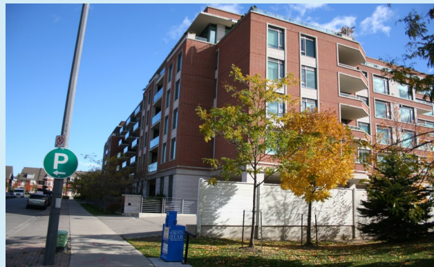
Figure B79 — Image of the Harbour Mixed Use Precinct
