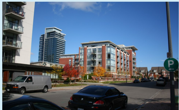
Figure B77 — Image of the Harbour Mixed Use Precinct
