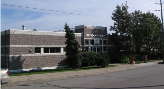
Figure B24 — Image of the Riverside Precinct
