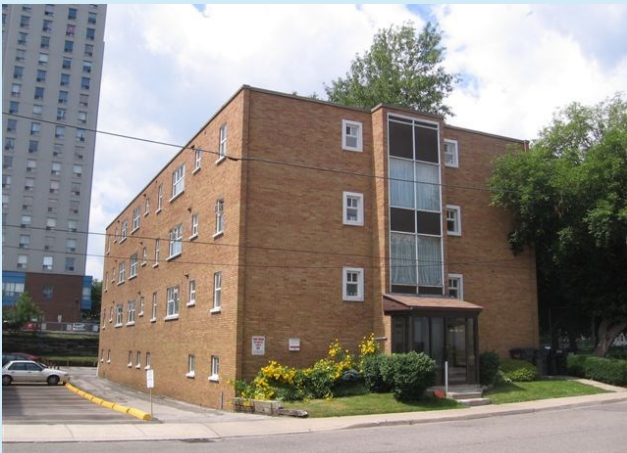
Figure B26 — Image of the Riverside Precinct
