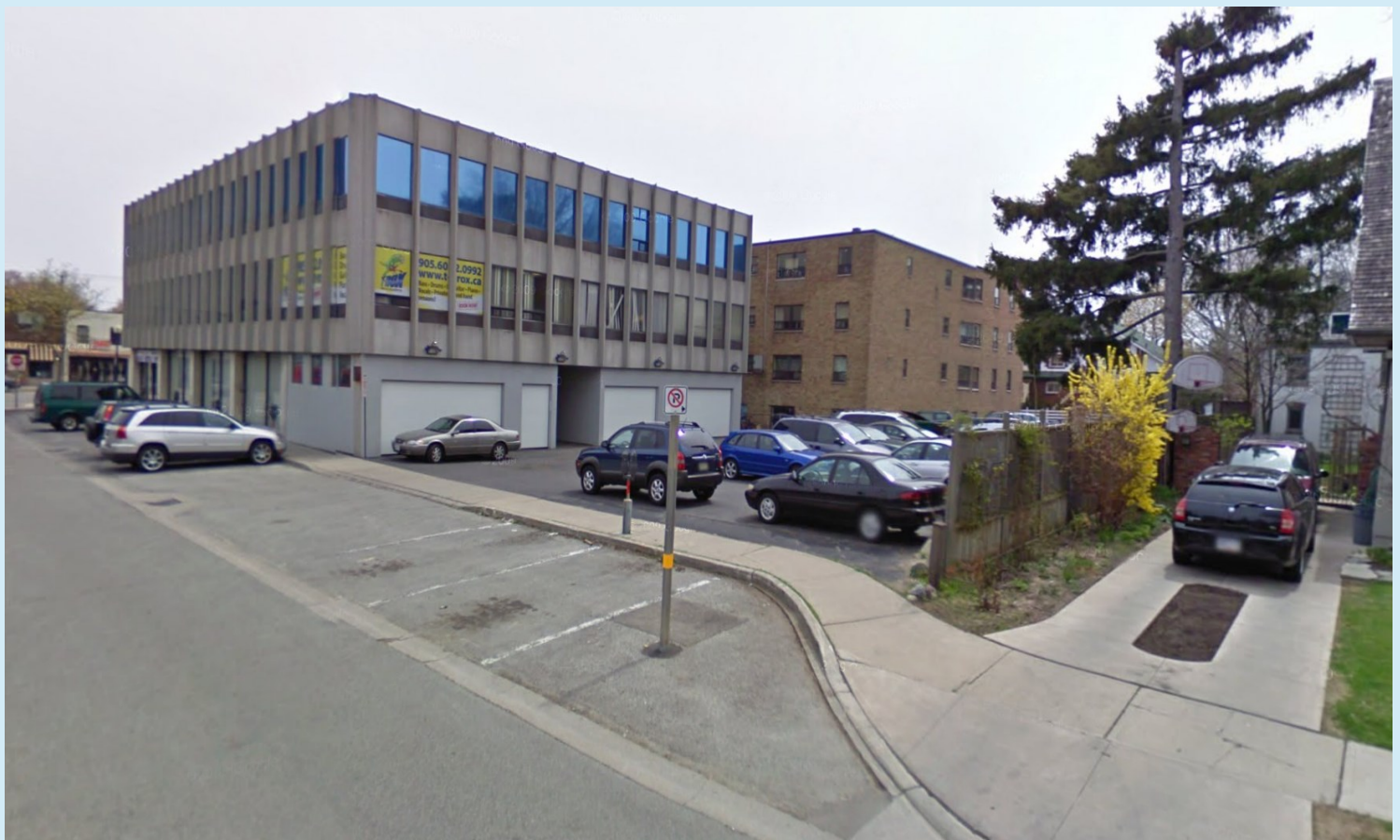
Figure C50 — Briarwood Avenue north of Lakeshore Road East
