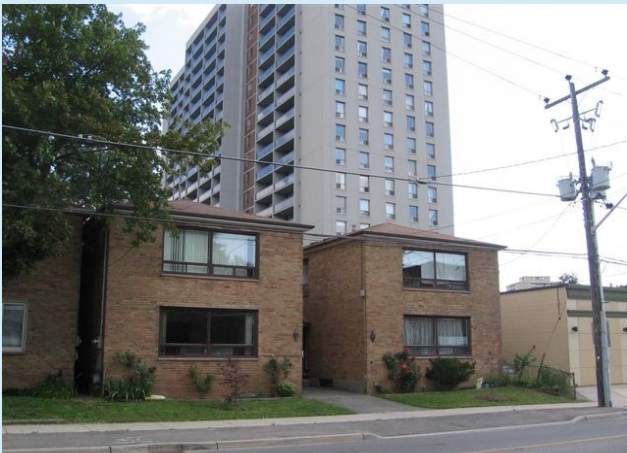
Figure B25 — Image of the Riverside Precinct
