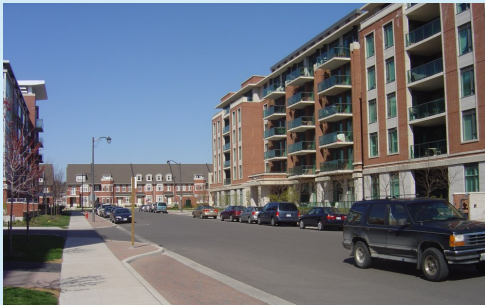
(top left) Figure B35 — Existing development south of Port Street East.
