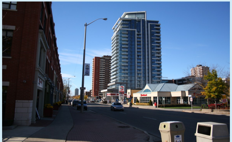
Figure B51 — View from Lakeshore Road East looking West
