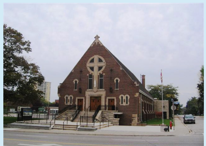
Figure B137 — 141 Lakeshore Road West, Designated
