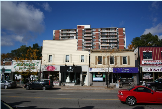
Figure B67 — Mainstreet building frontages
