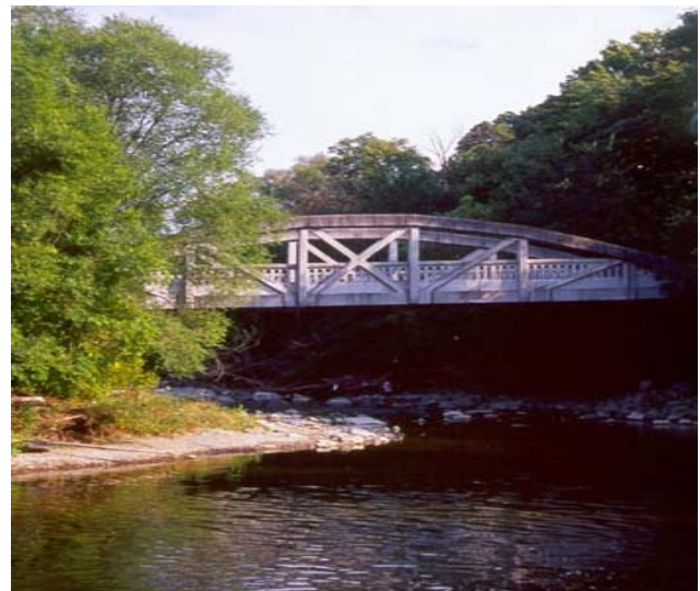
Figure 9-14: The Middle Road Bridge, located at the eastern end of Sherway Drive at the Etobicoke Creek, was built in 1909 and was the first concrete bow bridge of its kind in Canada.
