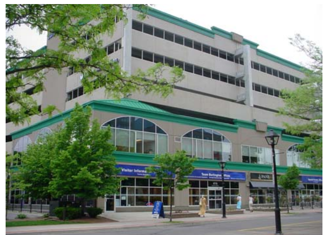
Figure 8-7: Parking garages are a better use of space than surface parking and provide an opportunity to incorporate a mix of uses, as this parking garage in Burlington illustrates.
