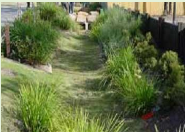
Figure B75 — Example of enhanced dry grass swale
