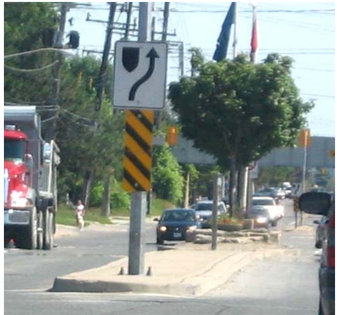
Figure 2-36 Current Median on Lakeshore Road West
