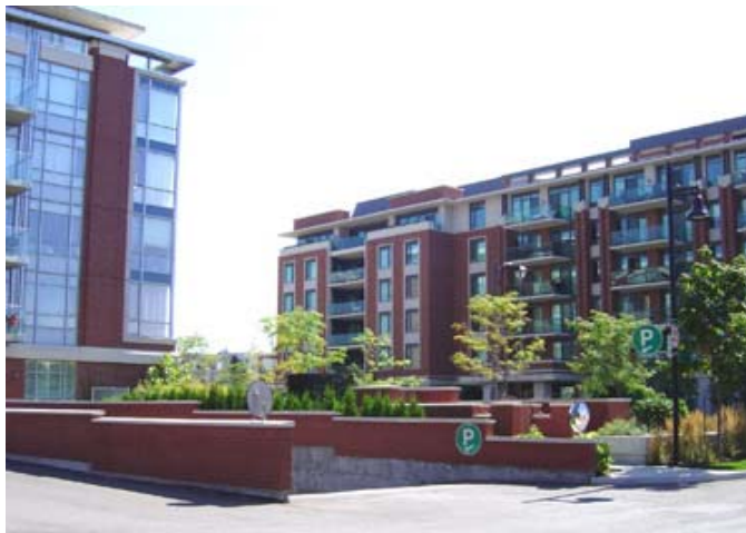
Figure 2-21 Underground parking Port Credit
