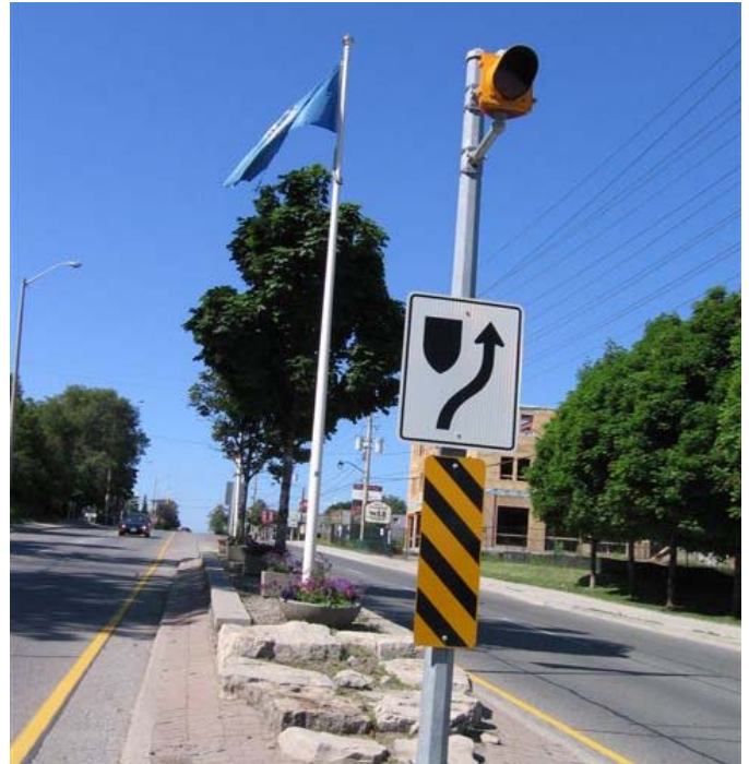
Figure 2-35 Current Median on Lakeshore Road West
