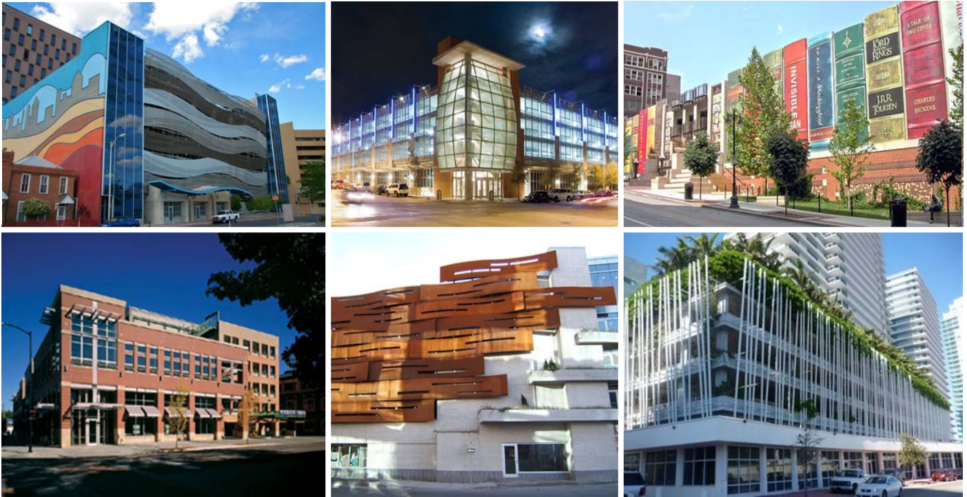
Figure 2-24 Different samples of façades that articulated with architectural treatment to mask structured parking.
