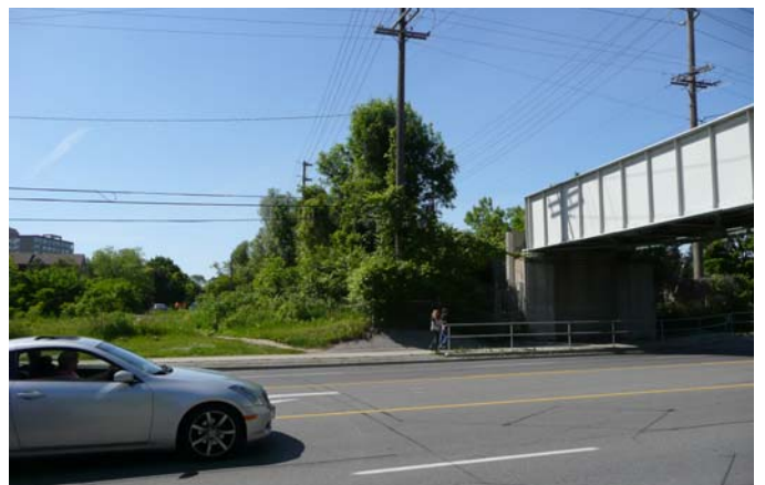
Figure 2-10 Rail Underpass on Lakeshore Road West
