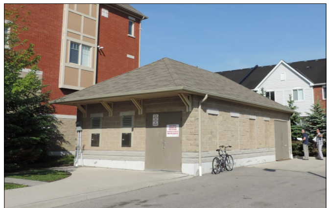
Figure 2.10: Waste collection and storage areas should be constructed of durable materials.
