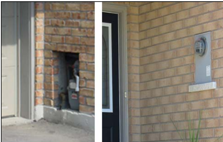
Figure 2.12: Place Hydro and Gas Meters and other utilities in concealed or recessed locations.
